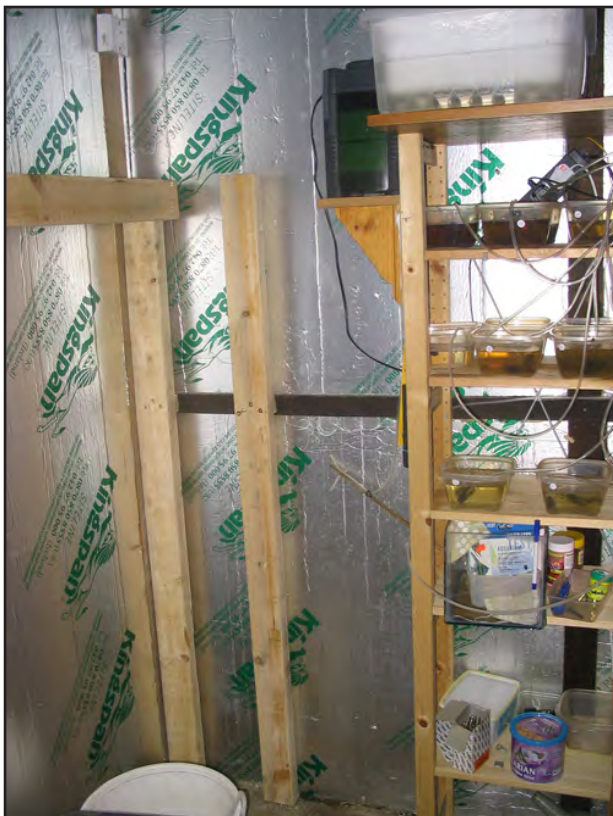
Stage 2 under construction
