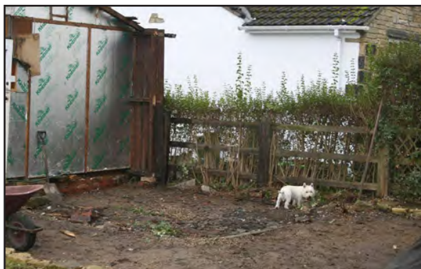
External insulation of the fishhouse (prior to demolition in 2011)
