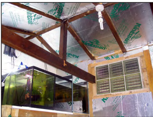
Ceiling, showing insulation
