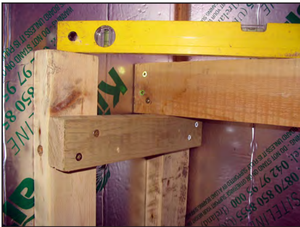
Detail of screw and cross brace support
